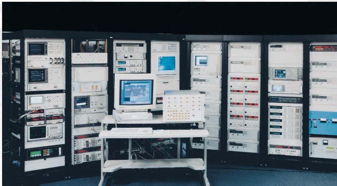
B2 avionics test bay subsystem
